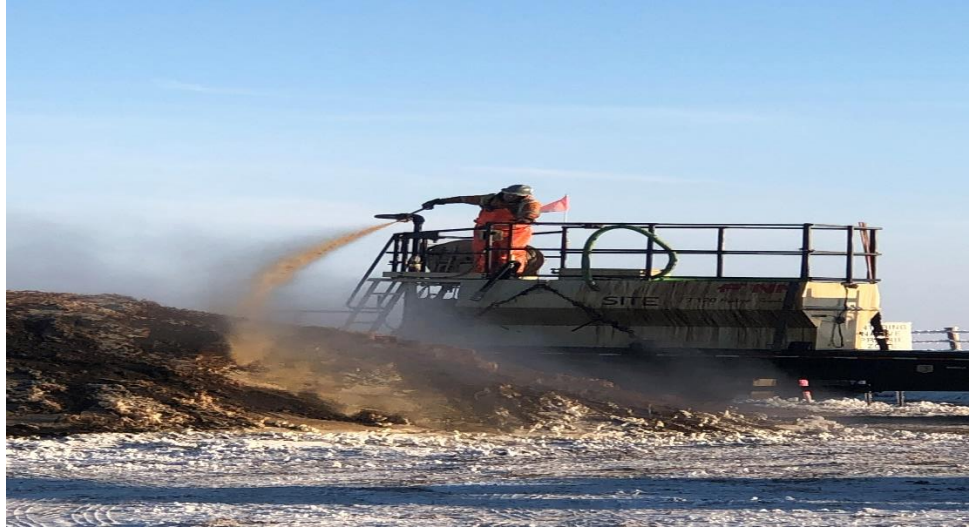
SPRAYING SOIL PILES WITH TACKIFIER.
