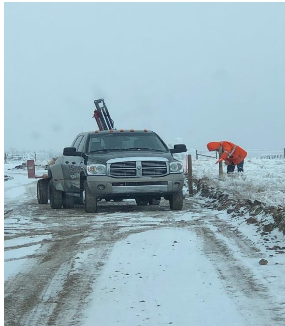
POUNDING POSTS AND REPLACING FENCE.
